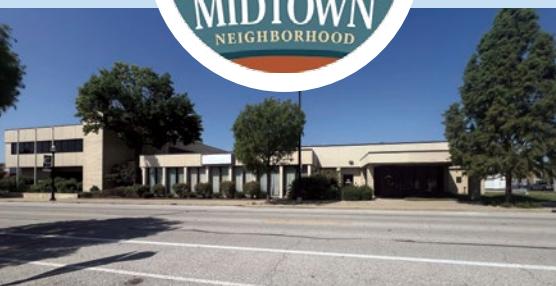
The Missouri Job Center will relocate to the three-story building at 1600 N. Boonville this fall. Read more on page 3.
